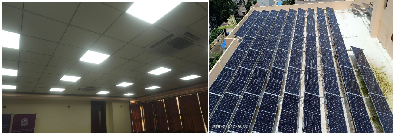
Image – LED lighting and solar energy installation
