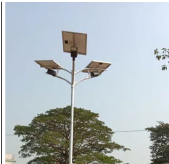
Plate 7.2.4.a Solar based street light
