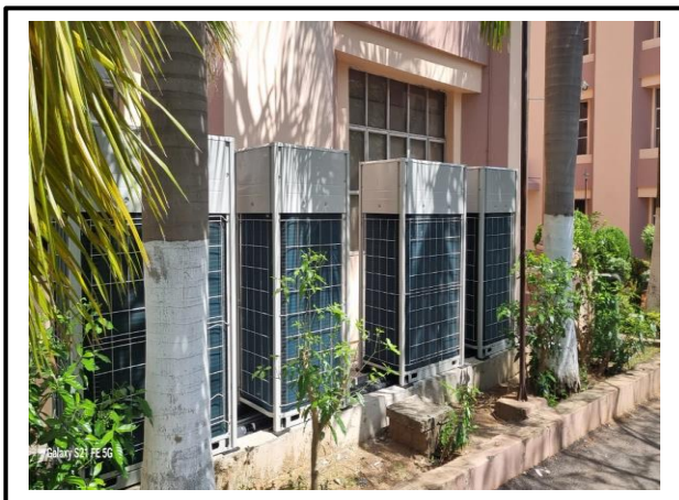
Plate 7.2.2.c. Centralized AC power consumption
