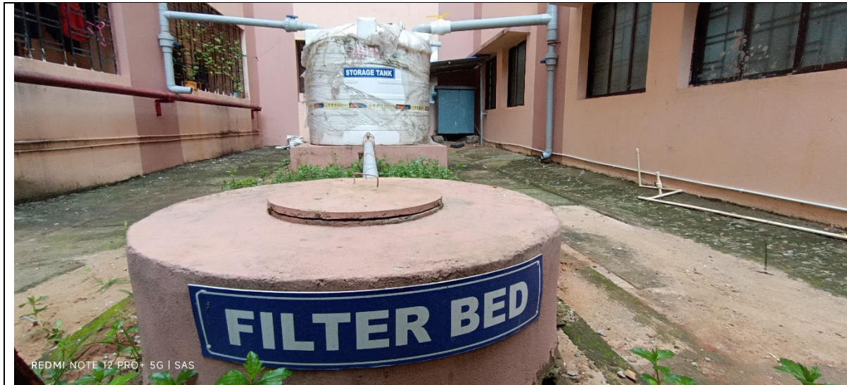
Plate 1- Rain water harvesting
