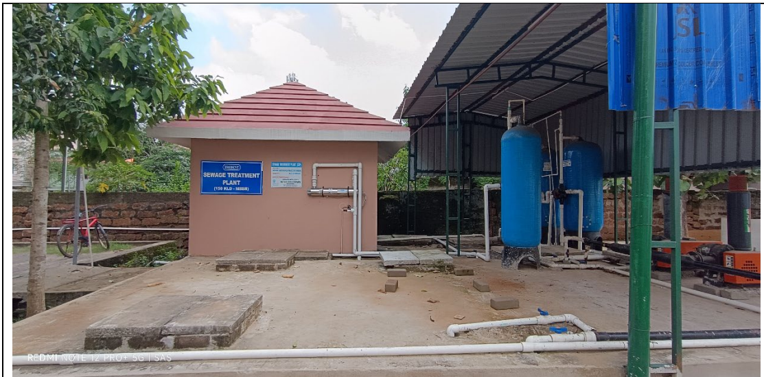
Plate 1- Sewage Treatment Plant
