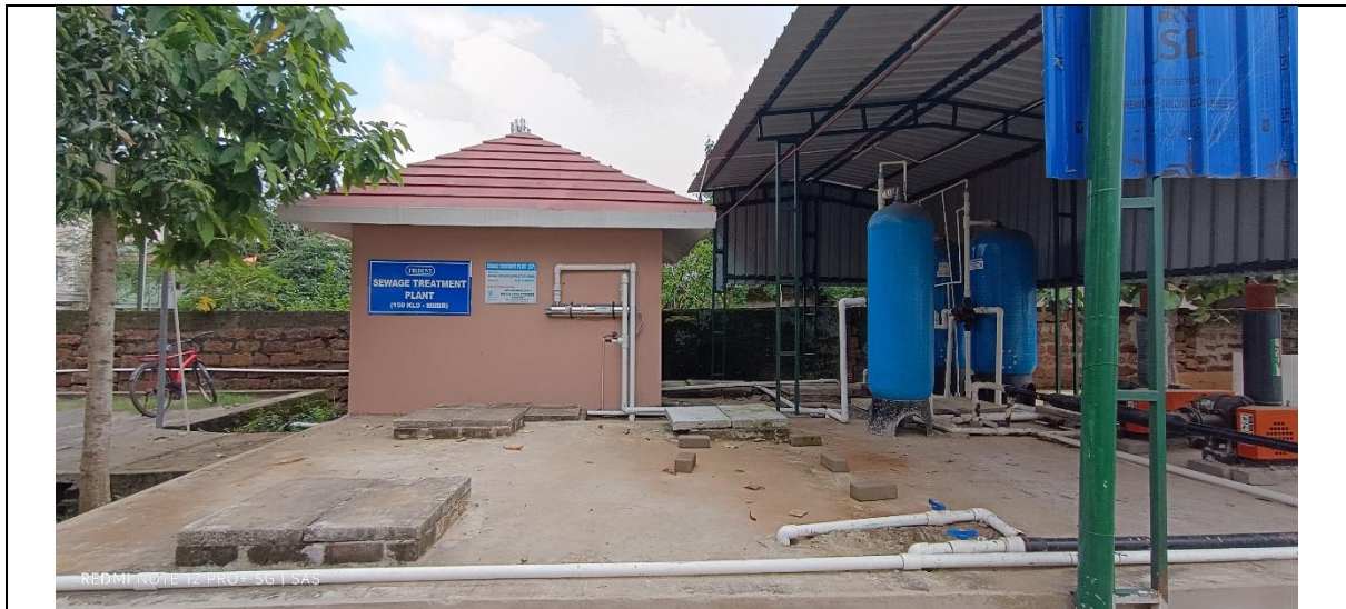
Plate 1- Solar powered 150 KLD (Kilolitres per Day) water treatment plant
