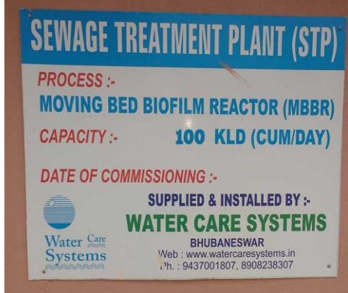
100 kLD STP plant
